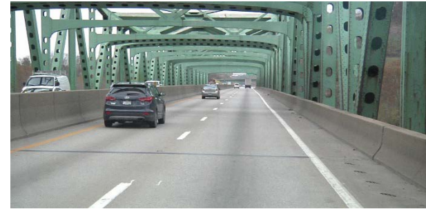
Bridge Deck (WV-I64)
