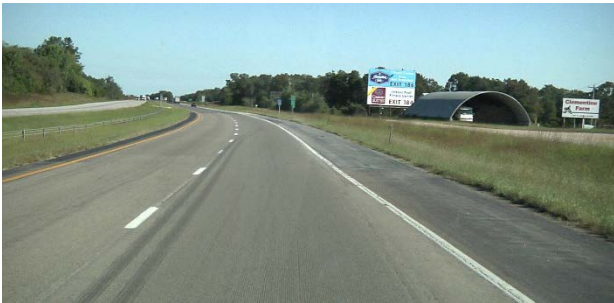
Grooved Flexible Pavement (MO-I44)
