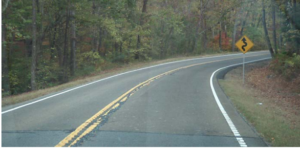
HFST Pavement (GA-140)
